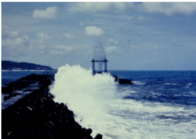
A power plant was built at the end of a breakwater. Working in the marine environment was very difficult.
