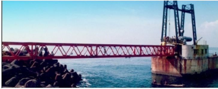
A bridge was built from the breakwater to the caisson.
