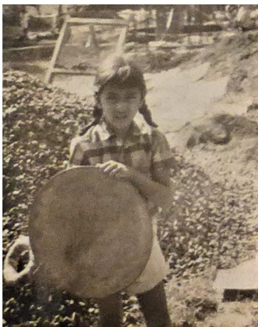
Devaki Bhaya, Director Sengupto's niece, assisting with the building of IIT Madras, c. 1965. Photo received from Devaki Bhaya
