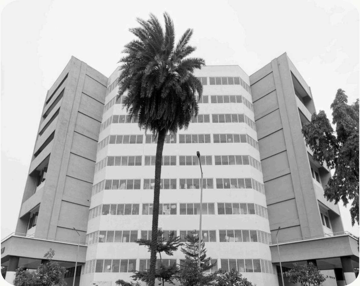
Below: A 100-year-old date palm preserved during the demolition of the old Mandakini and construction of the new 10-storey building.
