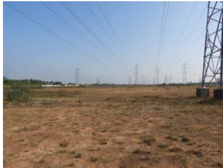
Electric transmission lines running through the campus.
