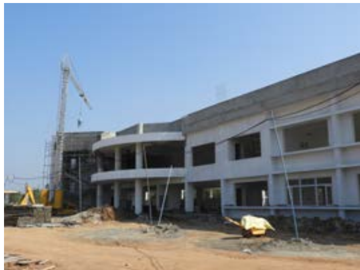
The National Technology Centre for Ports, Waterways and Coasts under construction.
