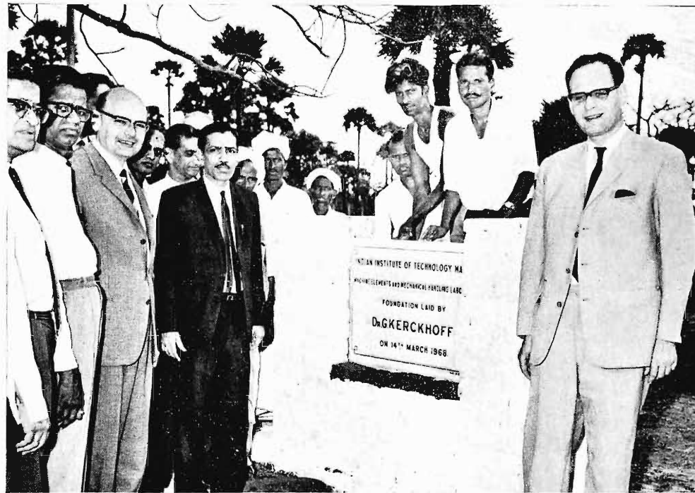
Dr. G. Kerckhoff, Minister for Economic Cooperation, Bonn, laid the foundation stone for the Machine Elements and Mechanical Handling Laboratory on 14th March, 1968
