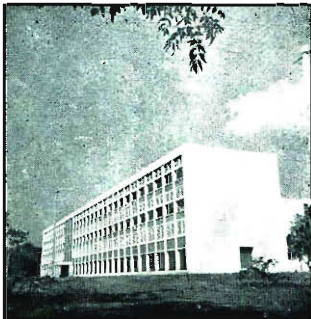
FROM A MILLION VOLTS TO A MILLIONTH OF AN AMP
